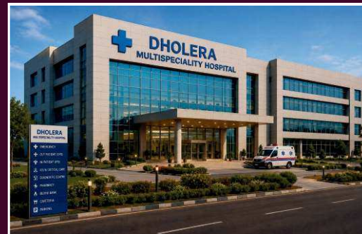
Dholera Multispeciality Hospital
